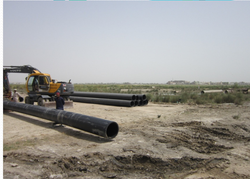
Pictures taken during laying of PE pipe at Qasimabad
