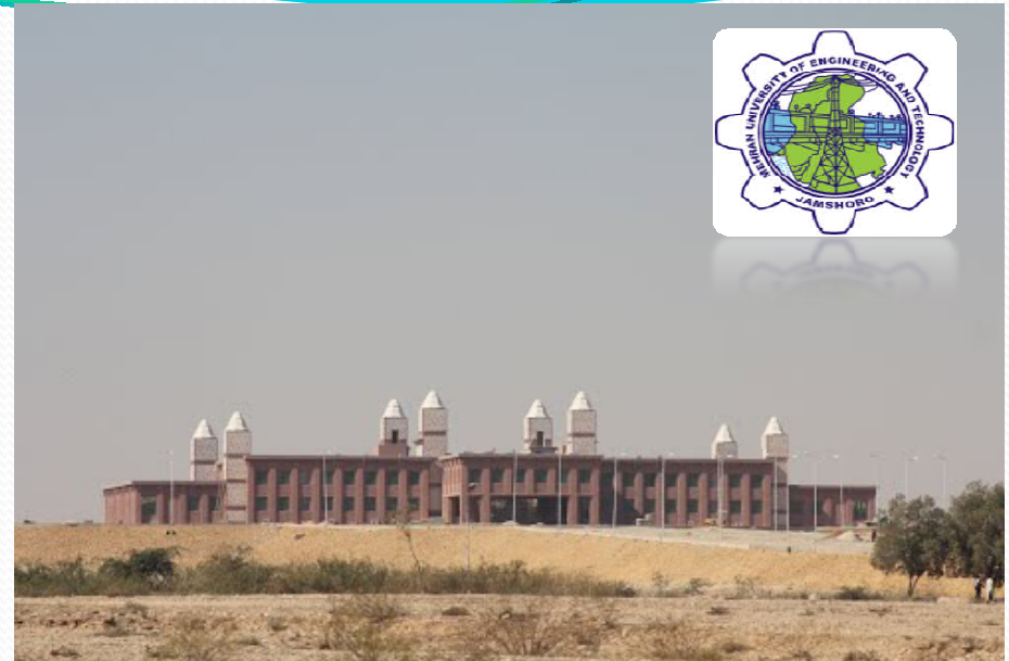
Administration Block MUET, Jamshoro
